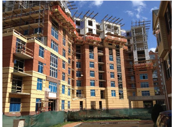
Figure 2: Site photo during construction
